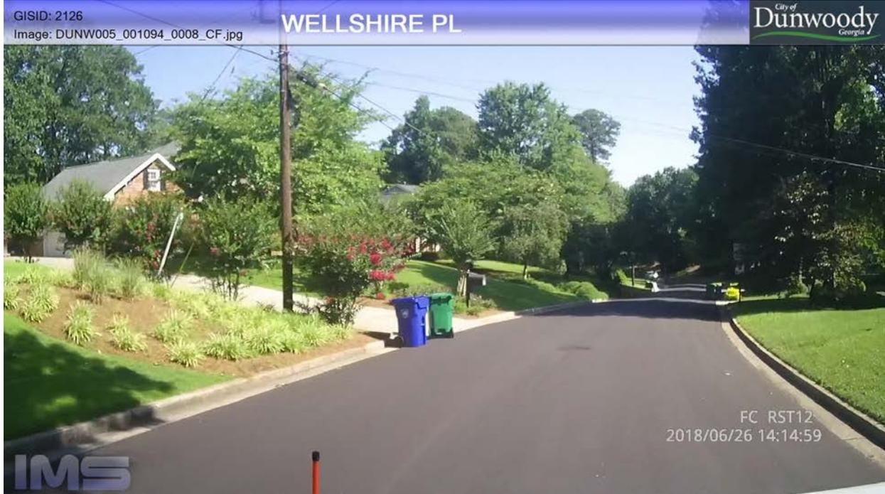
***Wellshire Place from Mount Vernon Road to Wellshire Lane (GISID 2126, PCI = 95) – Rated as Excellent, displaying little to no surface distresses. The ride is smooth and the surface is non-weathered and the base is strong. In a couple of years, this street segment would be an ideal candidate for routine maintenance activities such as crack sealant rehabilitation.***
