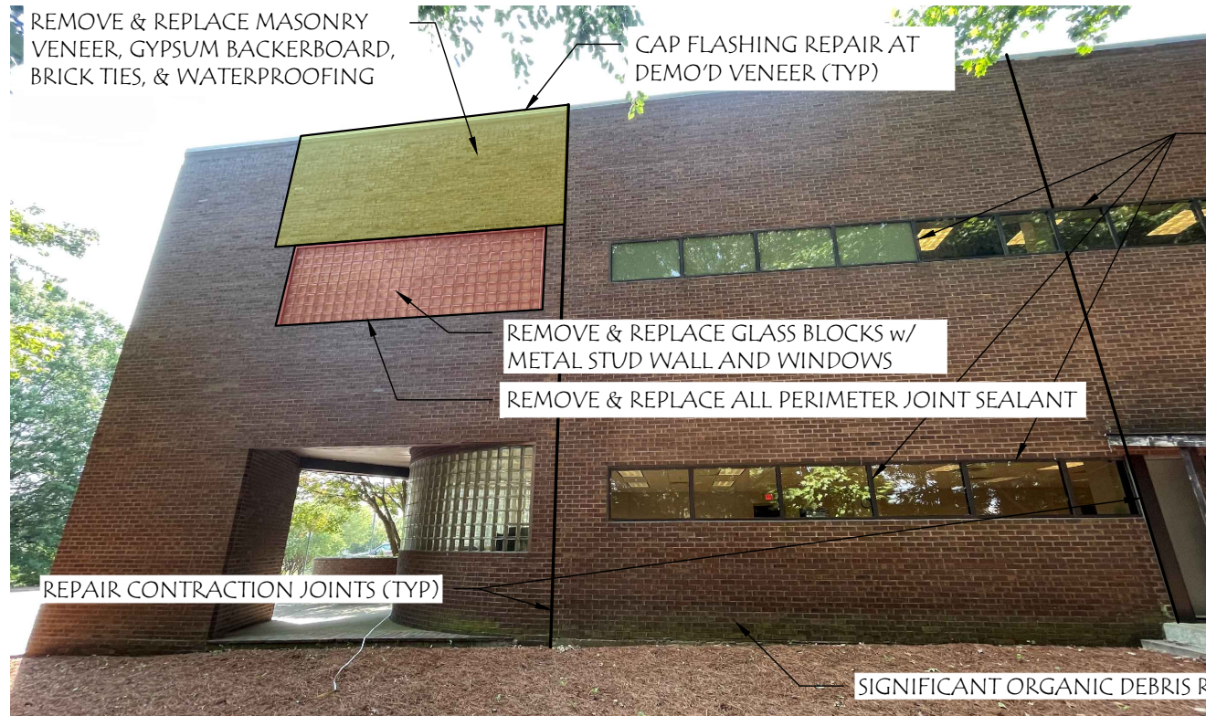
1 ELEVATION - PARTIAL NORTH WALL ELEVATION REPAIRS SCALE: NOT TO SCALE
