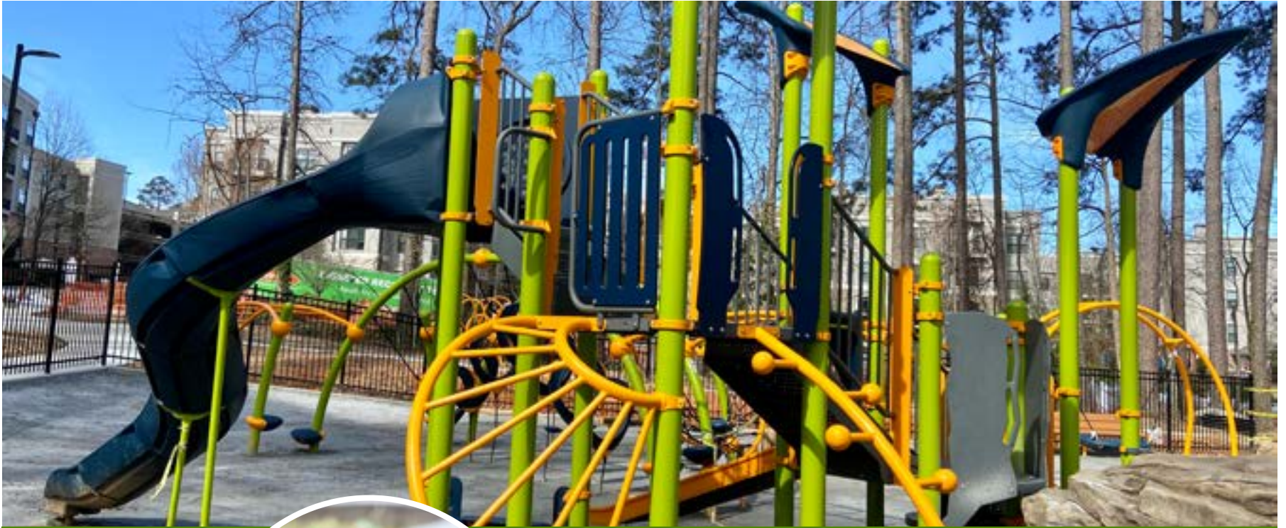
Construction completed on Two Bridges Park: Opening May 6
